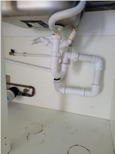
Photo 11 — Under kitchen sink
