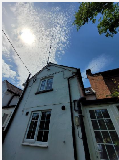
Photo 4 — Rear rainwater goods check
