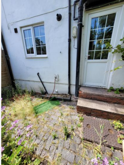
Photo 5 — Rear levels check
