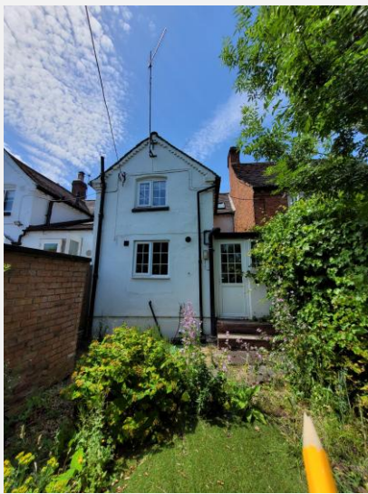
Photo 1 — Rear of property
