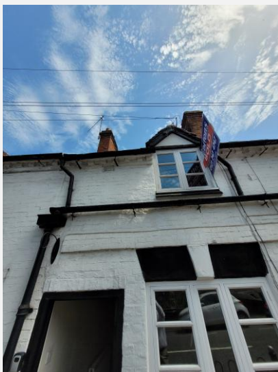
Photo 3 — Front rainwater goods check
